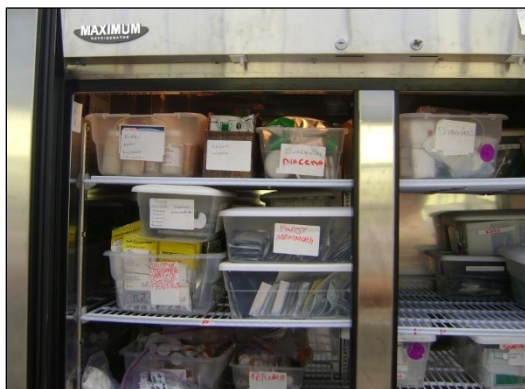
Most seed should be stored at 41 °F (~5 °C) and 25–30% relative humidity (RH). Commercial coolers/refrigerators are regularly used for seed storage but often do not provide sufficient humidity control to maximize seed shelf life. Tubs with lids can help to buffer changes in RH if your cooler opens regularly or other items share cooler space with stored seeds.
